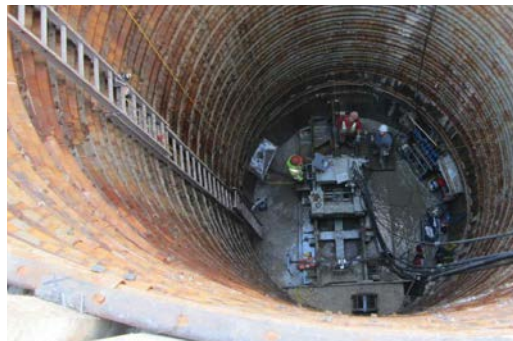
Construction crew working in 12-metre deep shaft near Shooters.
